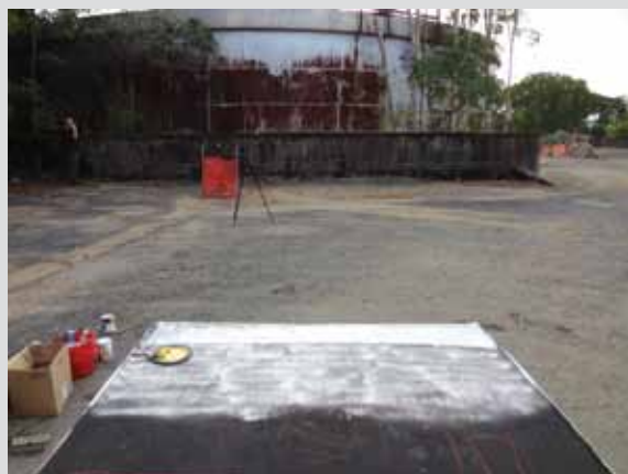
On site, oil tanks
